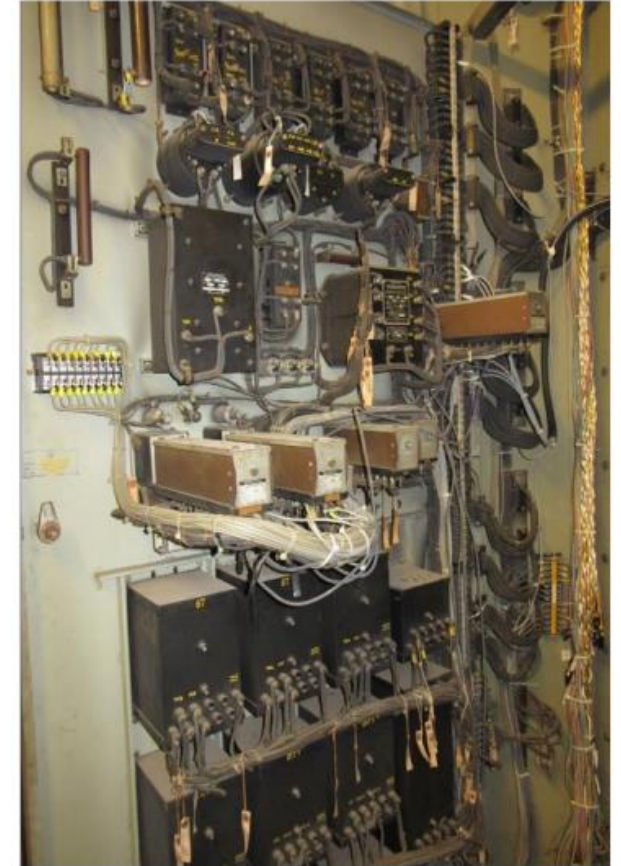
Figure 2: Wiring in Rear of Relay Panel [1]
