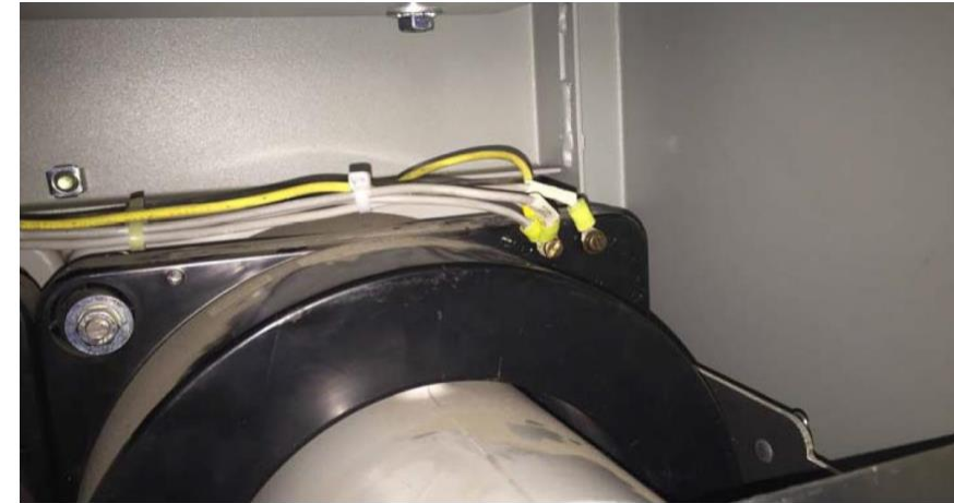
Figure 3: Added Neutral CT Connection to Complete 87N Circuit Post-Event [1]
