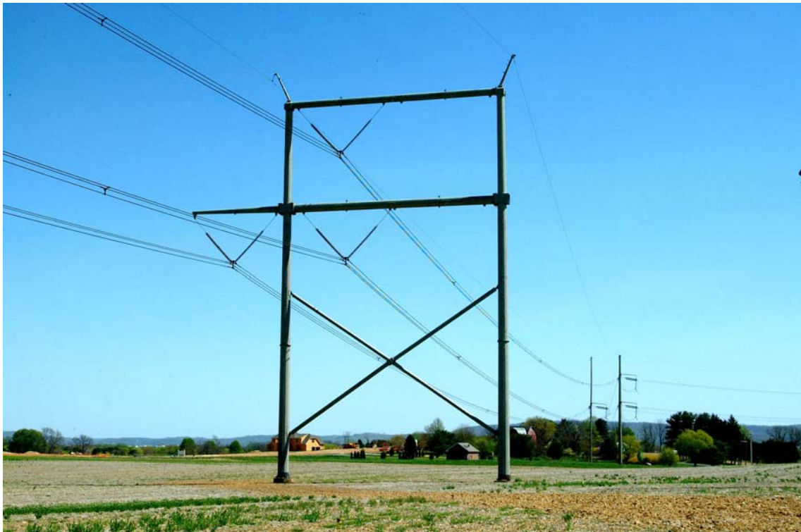
500 kV Double Circuit Construction, one circuit initially installed
