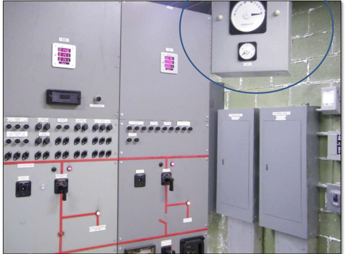
Control Panel with Synchroscope
