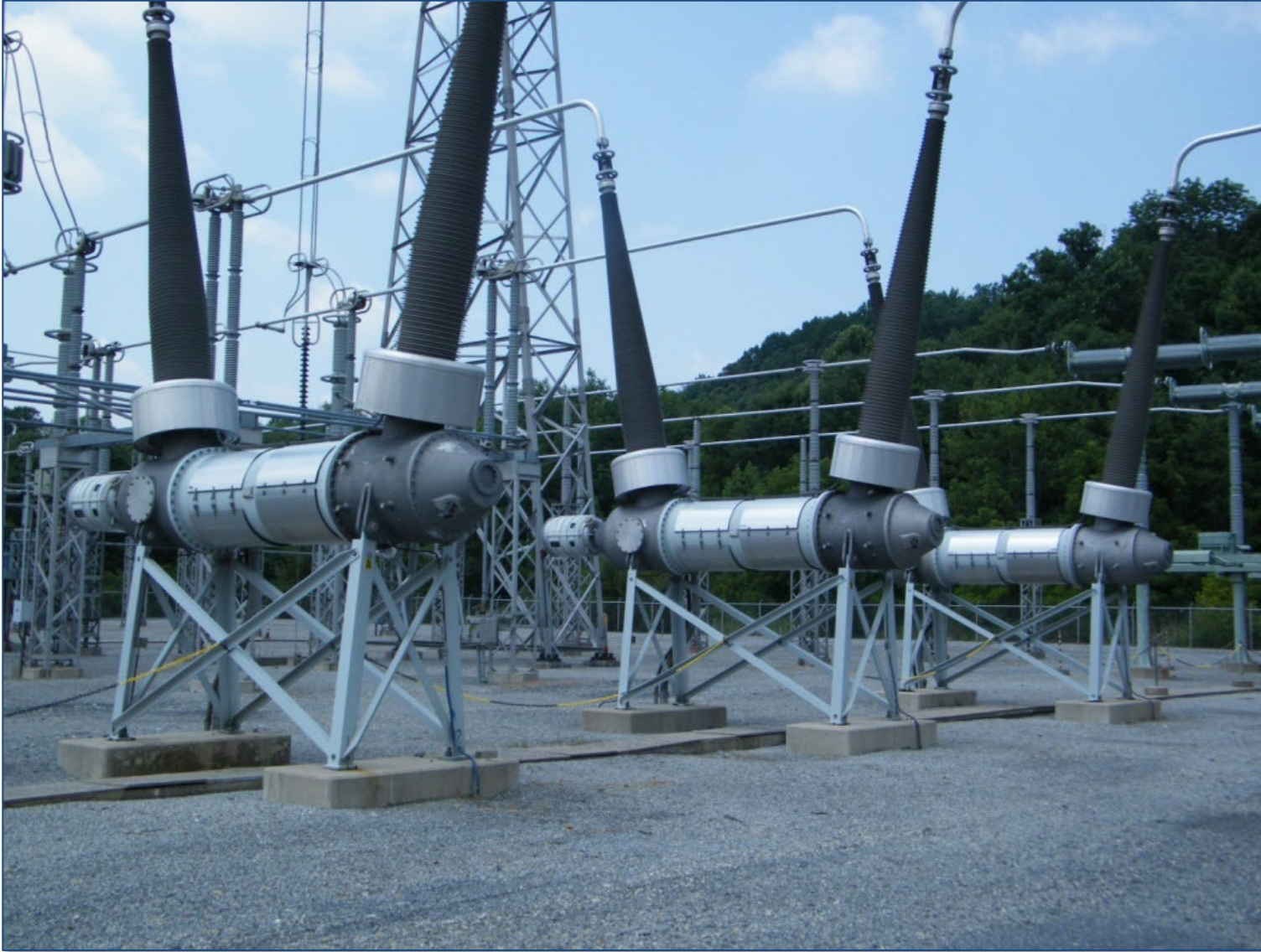
500 kV SF-6 Circuit Breakers
