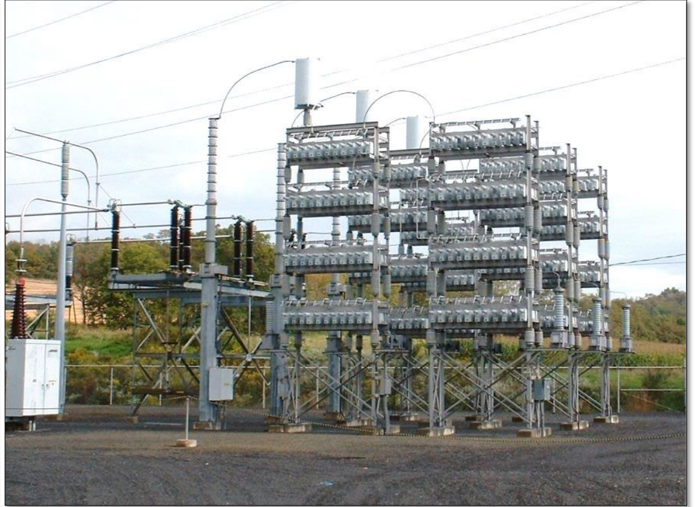
230 kV Capacitor Bank
