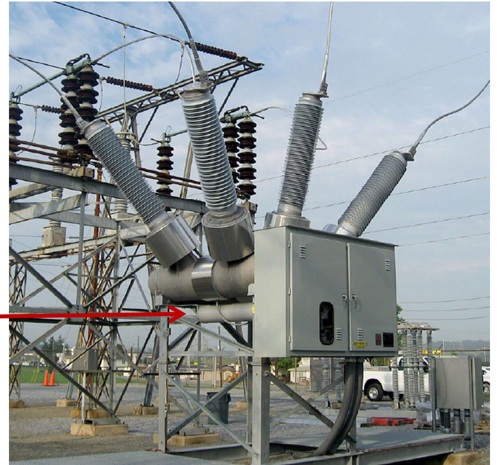
230 kV SF-6 Circuit Breaker →
