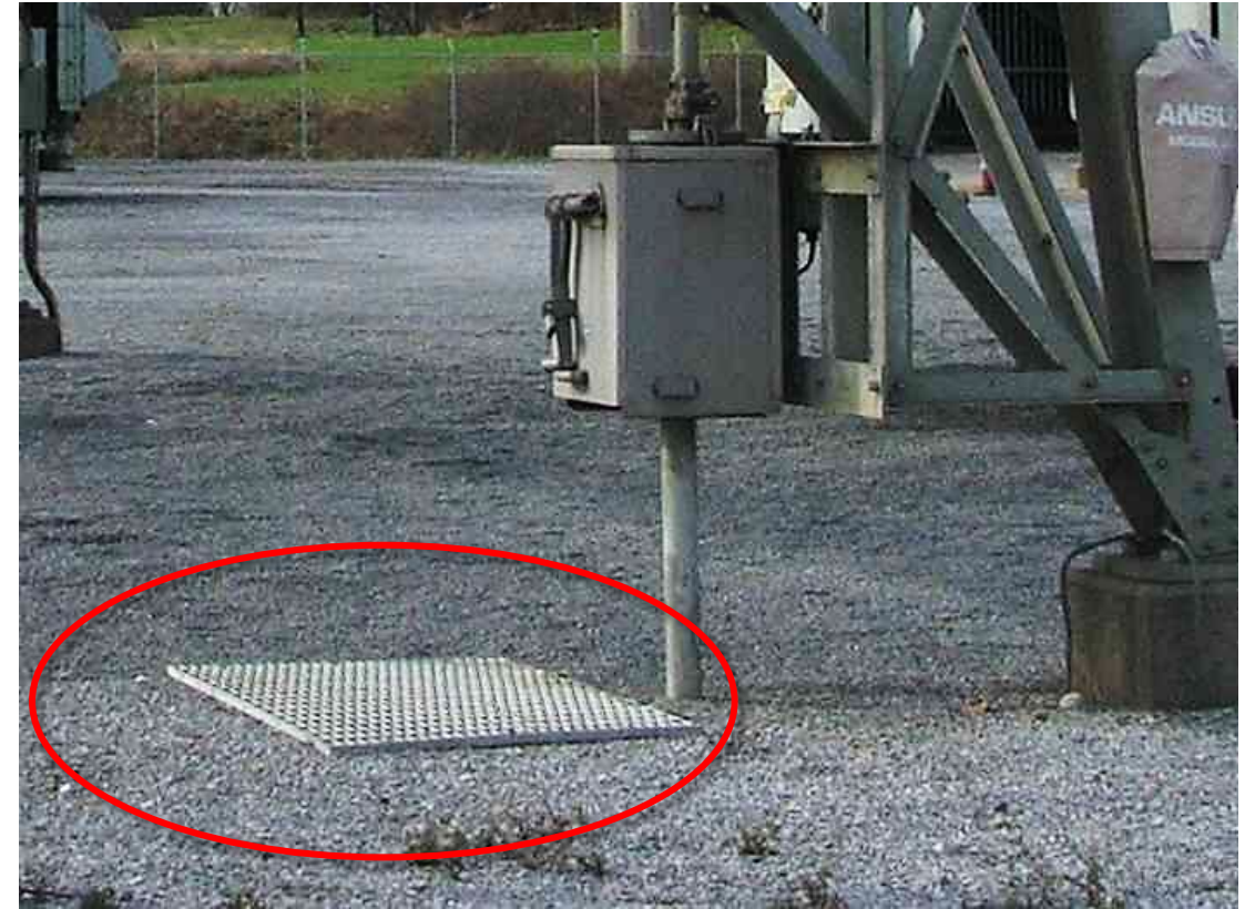
Grounding Mat Installed by a MOD
