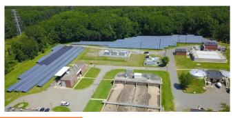
Caldwell Sewage Treatment Plant Supports Plant Operations Solar Facility: 902 kW-dc Battery: 1,000 kWh; EOS - Zinc Air
