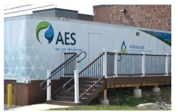
A two megawatt lithium-ion battery located at PJM's headquarters providing frequency regulation. Source:  $\mathsf{PJM}$
