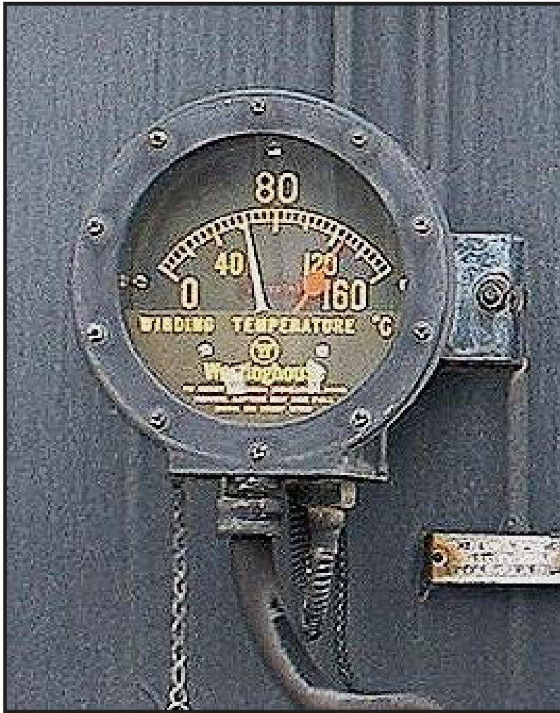
Illustrations of Analog Gauge Style Winding Temperature and Liquid Temperature Thermal Devices
