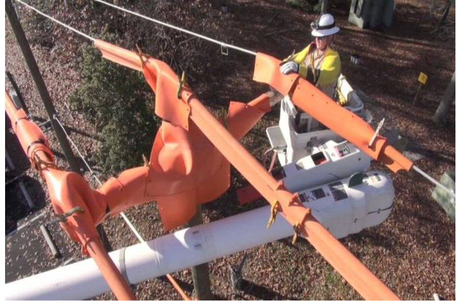
Effective Cover Up Performed on Overhead Lines (Dominion Energy Training Facility)
